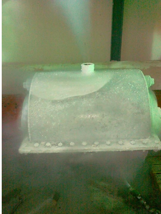
Pipe freezing jacket full of liquid nitrogen
