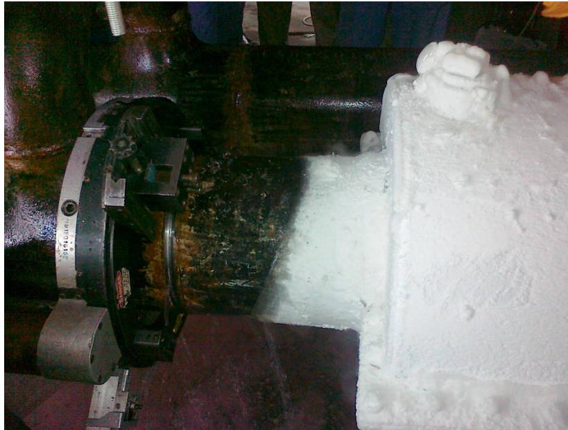
Used clamshell cold cutting machine for cutting and prepping the pipe
