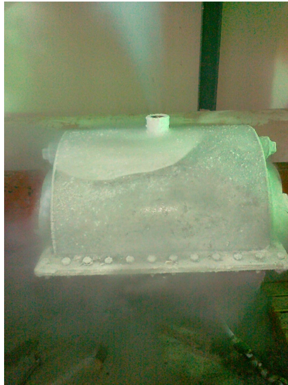
Pipe freezing jacket full of liquid nitrogen
