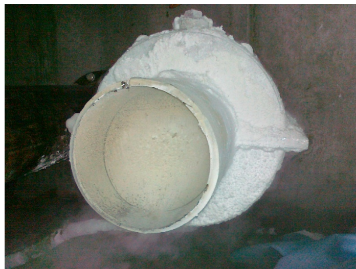
After the freeze, the pipe segment is cut, can see the ice plug
