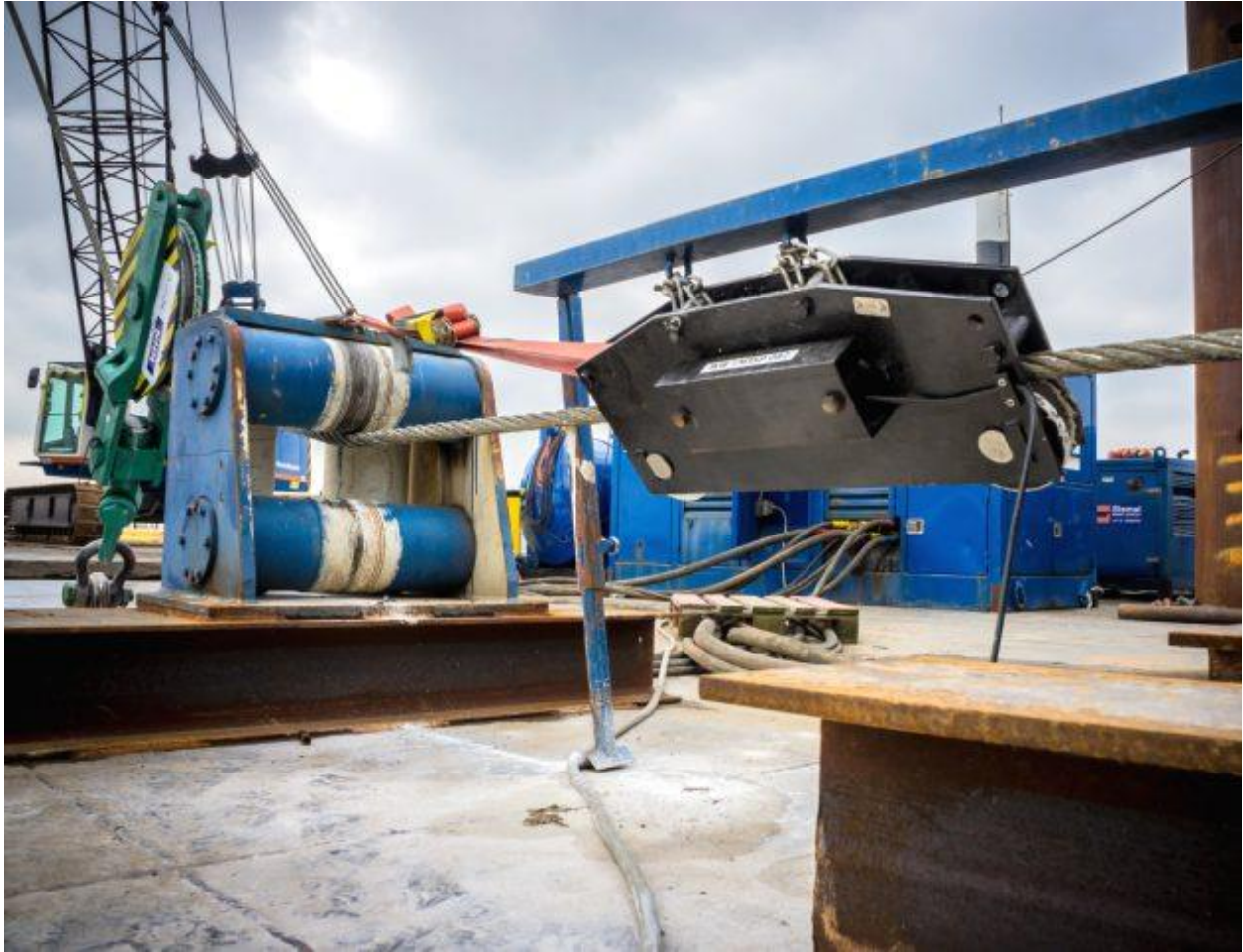
The load measurement system in use, during the cable lay.
