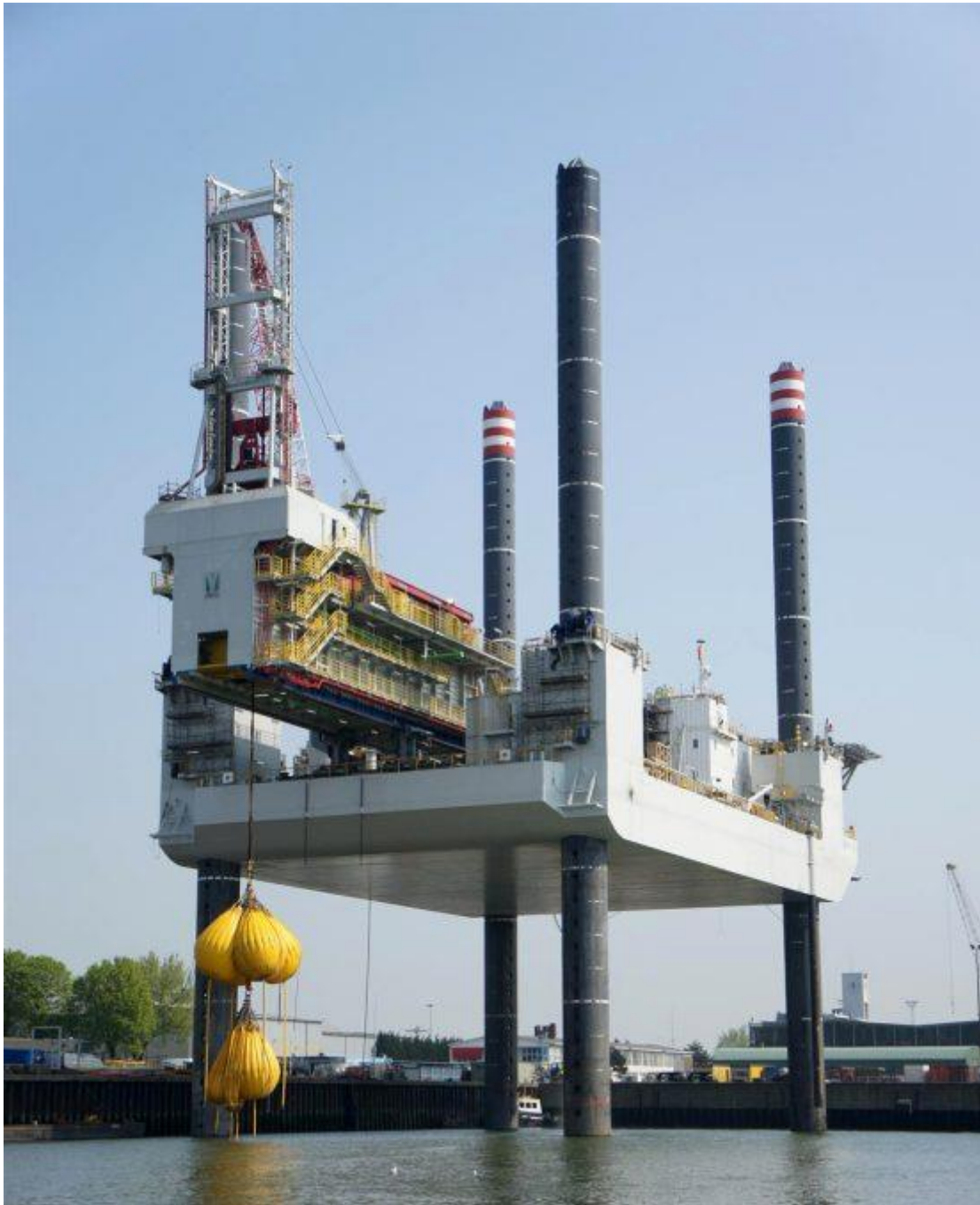
24-hour endurance test using 250 tonne proof load bags and a certified load cell on the cantilever system in an offshore drilling platform.
