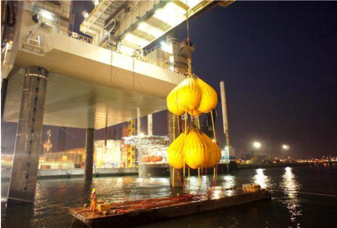
Water-filled proof load bags used in the endurance test
