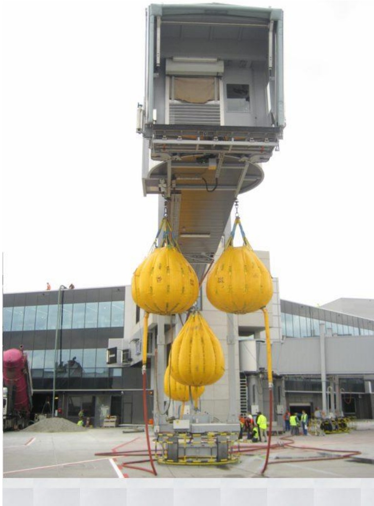
Water bags in use at the Frankfurt Airport
